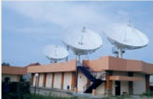
Backup Satellite Control Facility (BSCF), Bali
