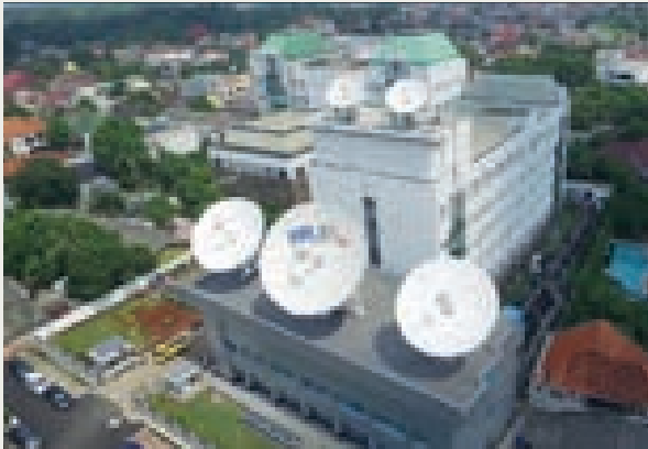
Primary Satellite Control Facility (PSCF), Jakarta
